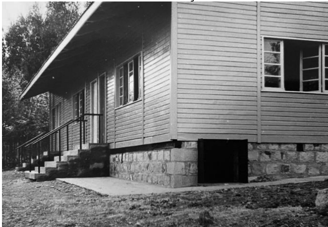
Laboratory Blocks at St. Joseph's School Campus
