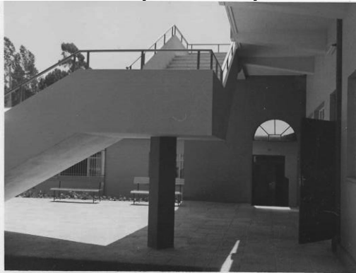
Staircase Detail, St. Mary's School study block
