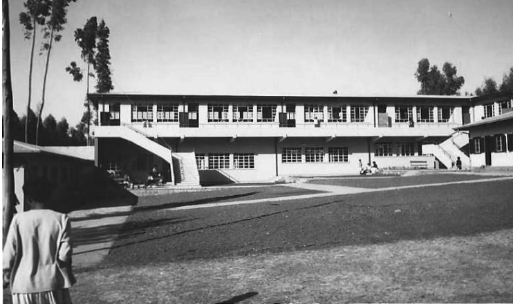
Lazarist Mission St. Mary's School study block overall view
