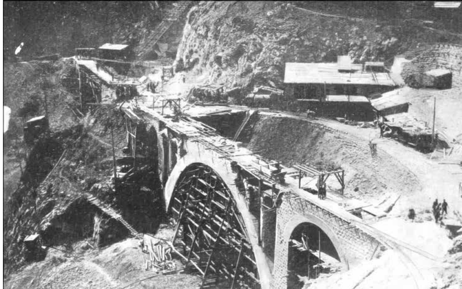
Baghdad Railway construction on the Taurus mountain 1912-1915 - Source Bill Milhomme
