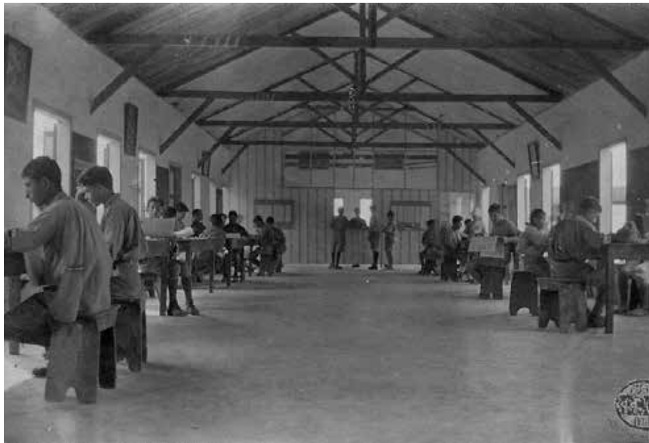
The library and reading room at Jbeil Orphanage
